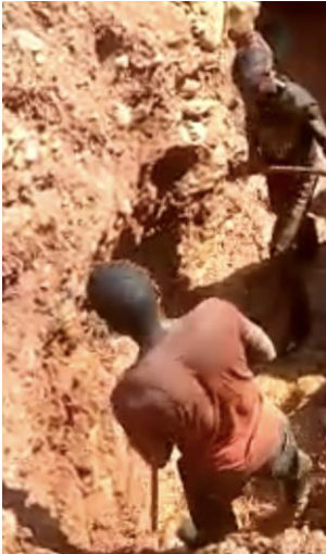
Hand digging, spade
